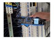
Set the switch to AUTO, connect and read the values directly. Shows current and voltage together.
